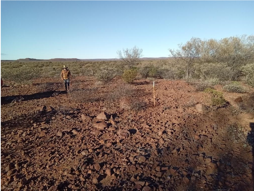
Figure 3. Preparing drill sites at the Mount Vernon Project.
